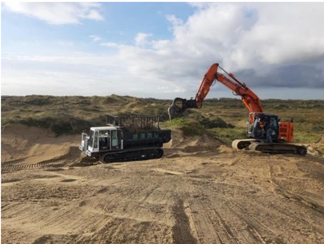
Figure 19: The excavator and the tracked dumper during the works in the Westhoek nature reserve ( © Reinhardt Strubbe ).
