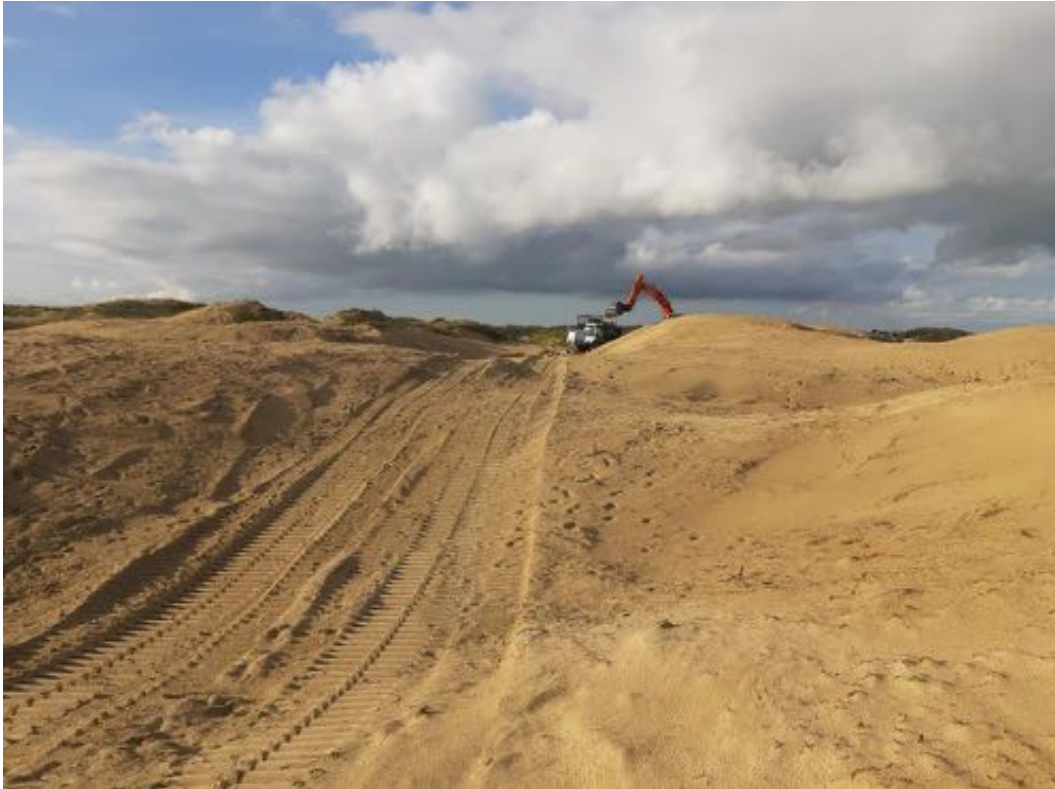
Figure 18: The excavator at work in the Westhoek nature reserve ( © Reinhardt Strubbe ).
